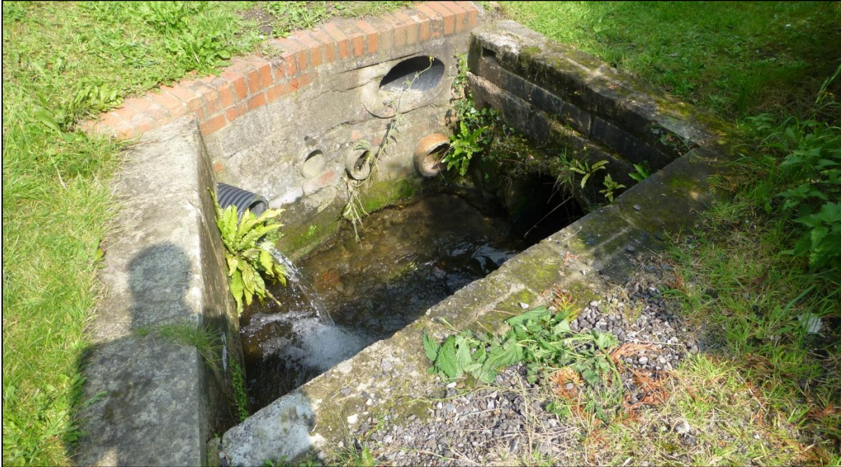
Figure 10: Drainage Outfall near Spring Cottage
